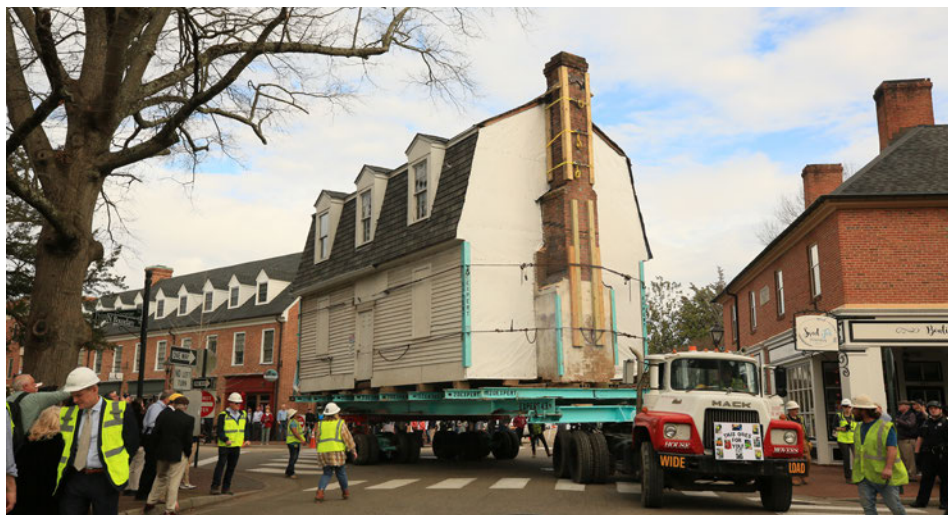
The Williamsburg Bray School building was relocated from its location on the W&M campus to its permanent home in Colonial Williamsburg at Francis & Nassau streets. (photo by Stephen Salpaukas)
